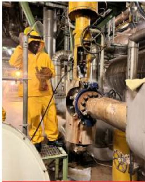
DURING ONLINE LEAK SEALING
