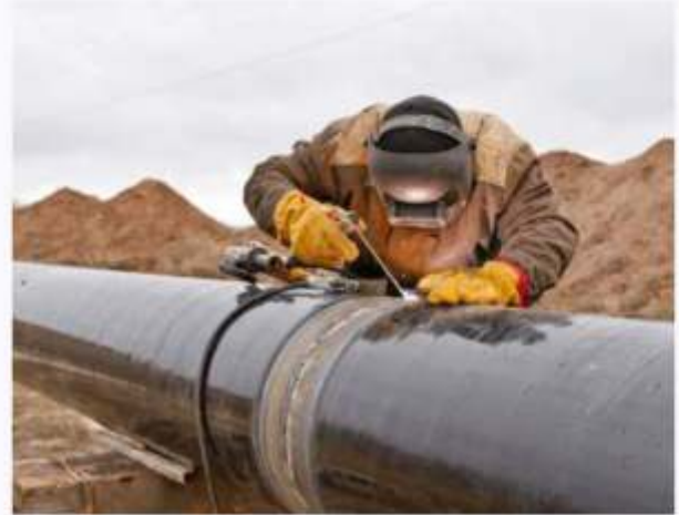
Pipeline Installation & Steel Fabrication
