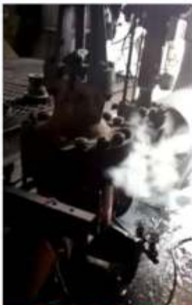
FLANGE JOINT LEAKAGES
