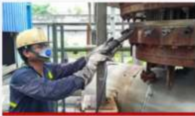
ONLINE LEAK SEALING
